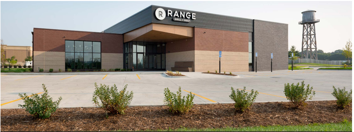
Slingshot defined the restaurant and entry area with changes in masonry color and patterning.
